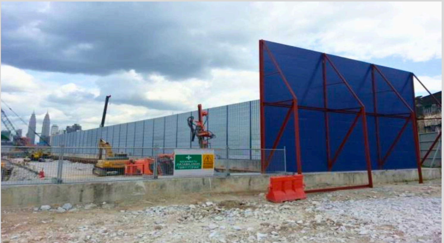
After Installation of Temporary Noise Barrier
